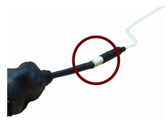
2. Peel plastic liner off Butyl Rubber Fusion Tape.
